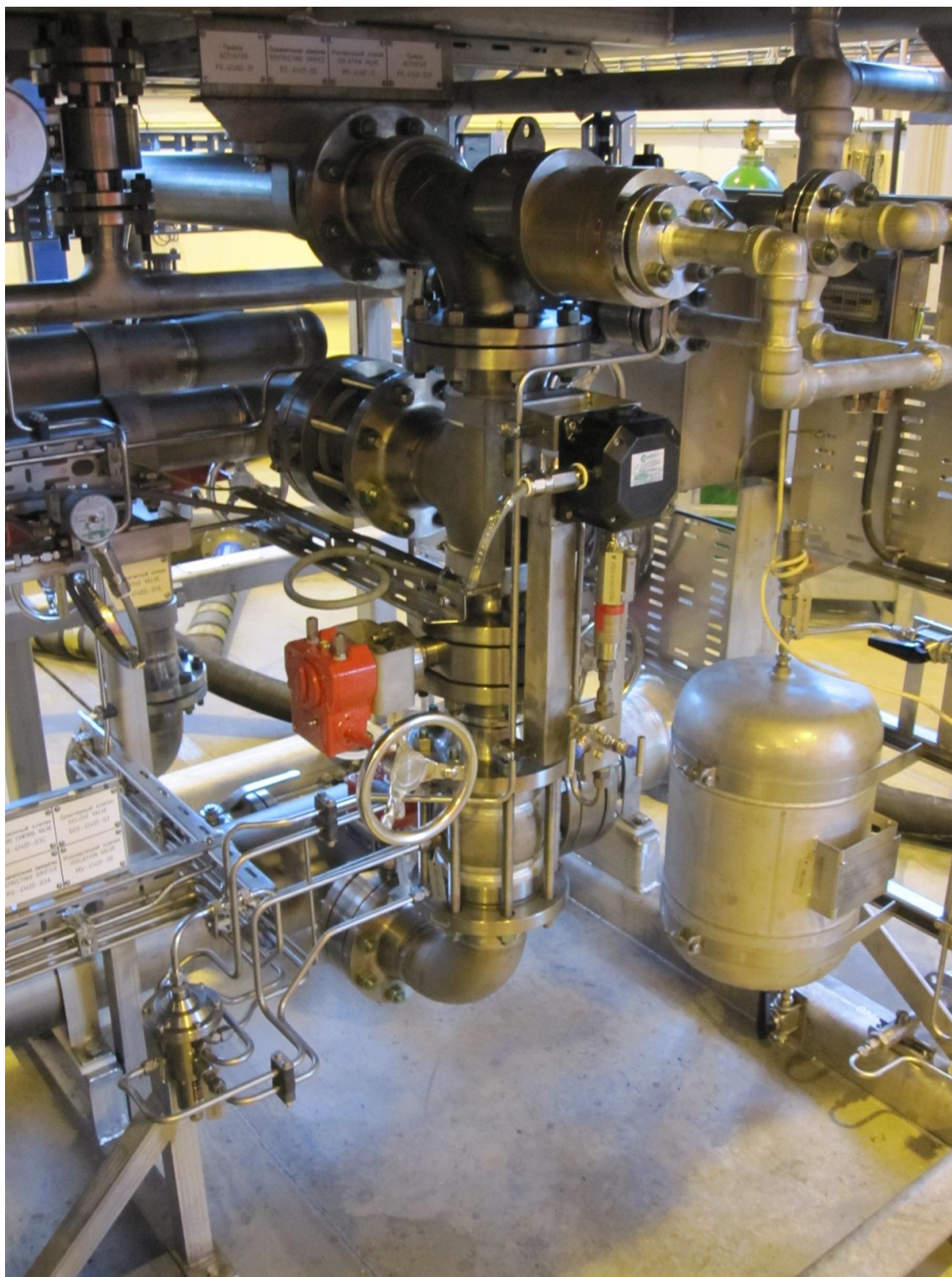
Figure 14: Inline Foam Turbine Pump Proportioner
